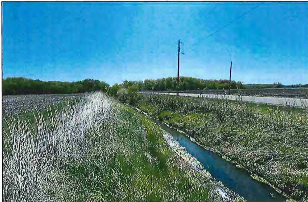
Photo pt 0014: East-west lateral ditch along 143 rd St. NE (facing east)
