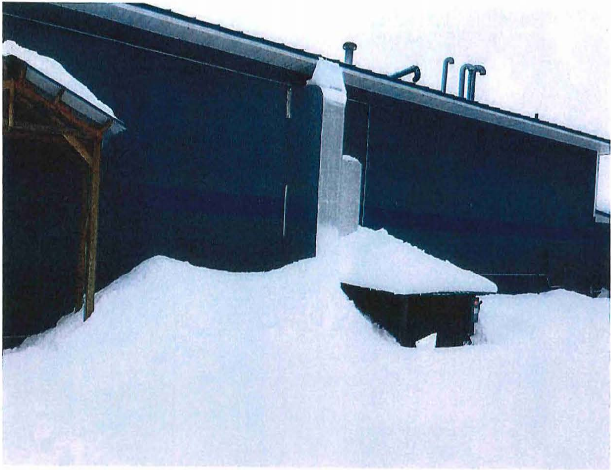
Canopy and HVAC southeast
