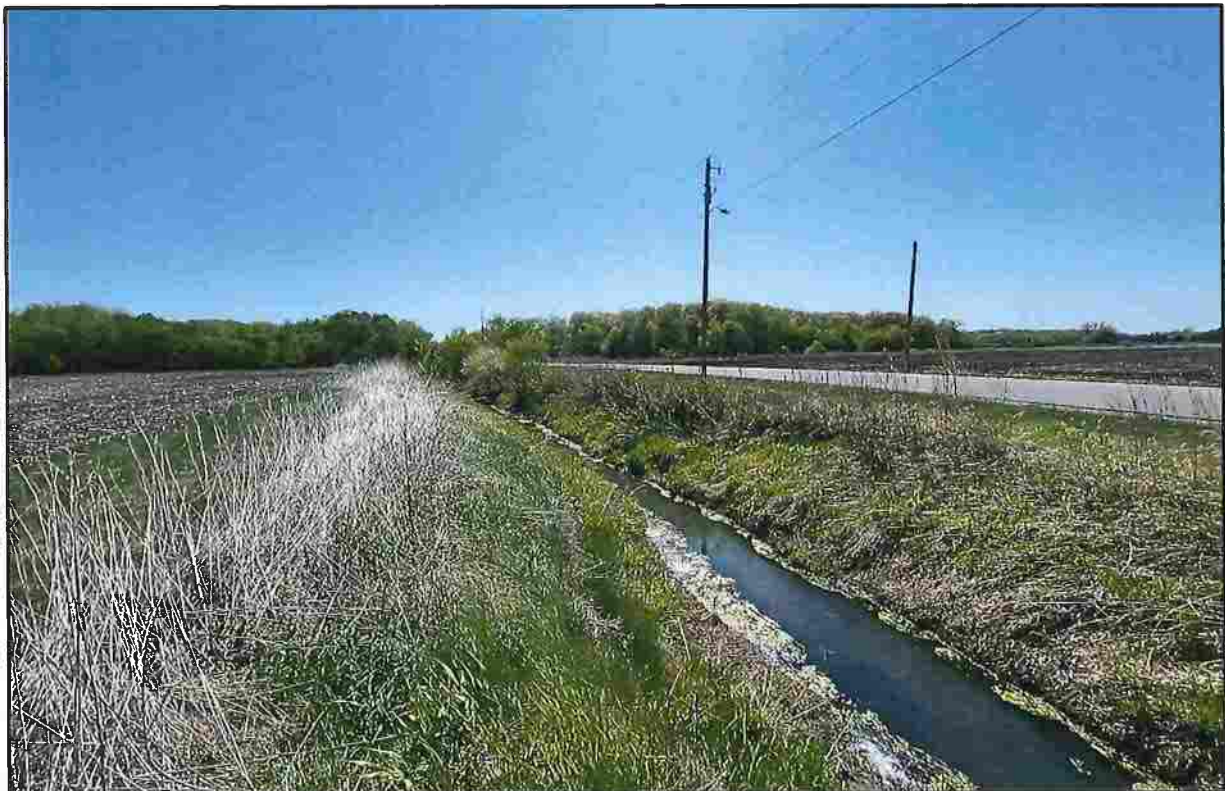
Photo pt 0014: East-west lateral ditch along 143 rd St. NE (facing east)
